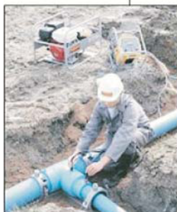
ELECTROFUSION OF 90° SPIGOT ELBOWS (2 BASES 1 T' CONNECTOR)
